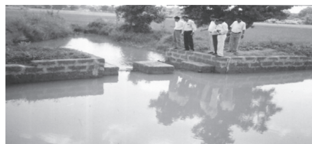
Fig. 5. Check dam for groundwater recharge
