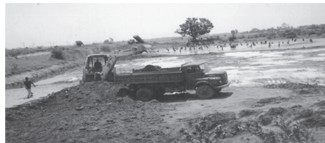
Fig. 4. Preparatory work for construction of check dam
