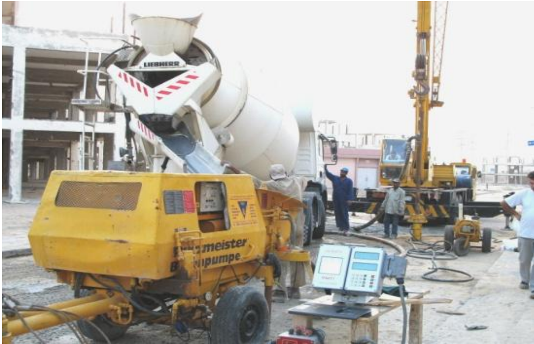
Figure 2: Delivery of cavity filling mix
