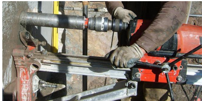
Figure 5: Extracting a concrete sample from a pier of Ghotour railway bridge
