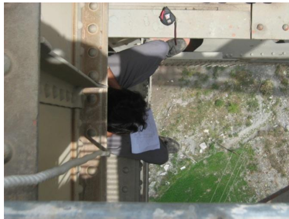
Figure 6: Preparing as built plan of Ghotour railway bridge
