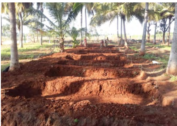
Plate 1. Preparation of pits
