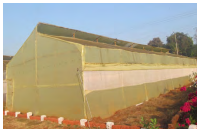
Fig. 1. Naturally ventilated bamboo polyhouse constructed at Dapoli (Konkan region, India) (Source: Jadhav and Rosentrater, 2017a).
